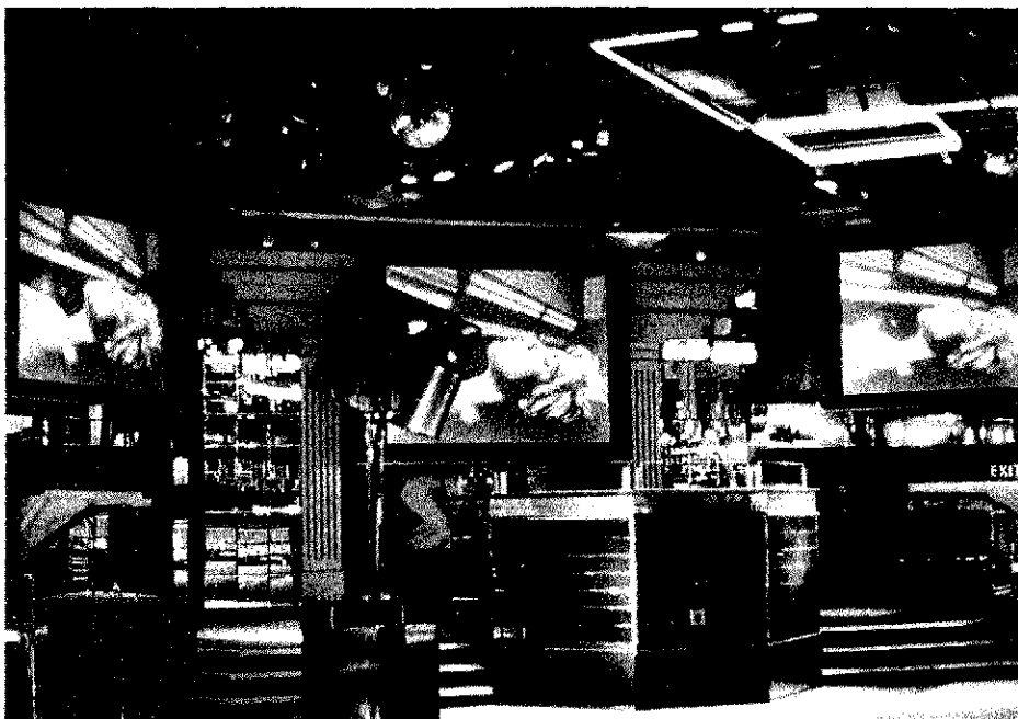
Amark's five projector installation at Busby's, Charing Cross.
